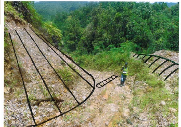
➤ Slope trimming & cut-off drains.
